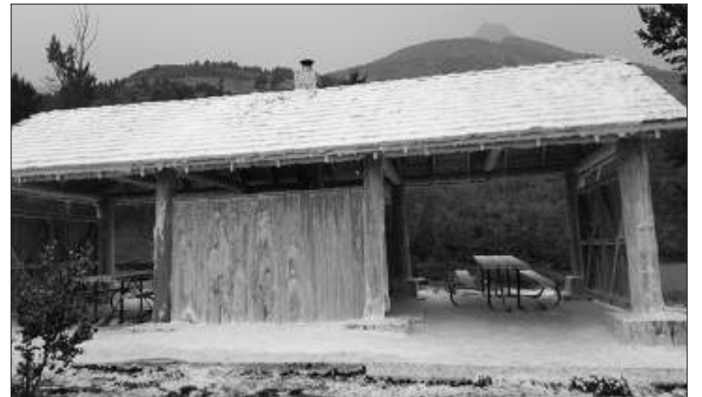
Picnic shelters within Waterton Lakes National Park sprayed with a biodegradable fire retardant foam to help protect from the growing flames.
